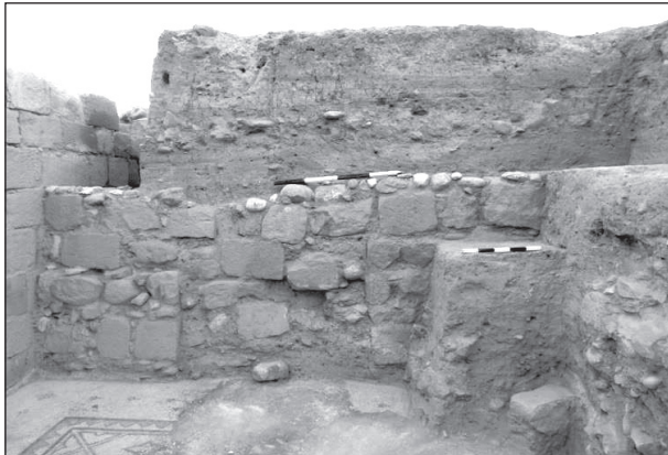
9. West section of Trench IX, showing the original west wall of the church, the later-phase wall built on top of it, blocking the west doorway from the outside (R. Schick).
